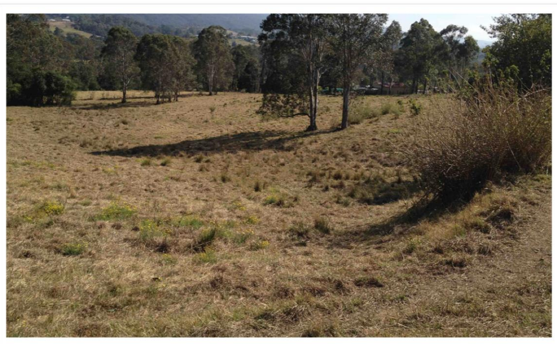
Figure 6: Dam Overflow path
